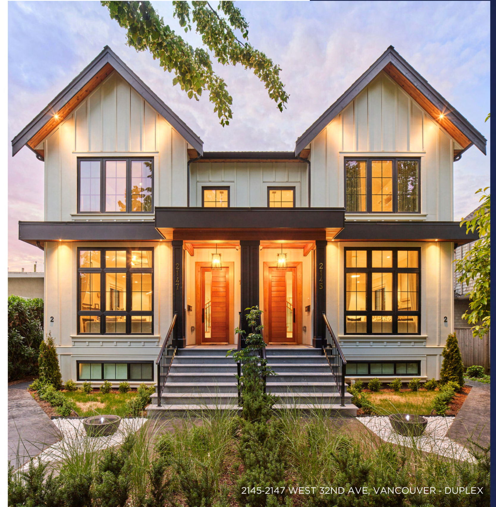
Quilchena Farm House "It Takes Two" Multiplex Project
